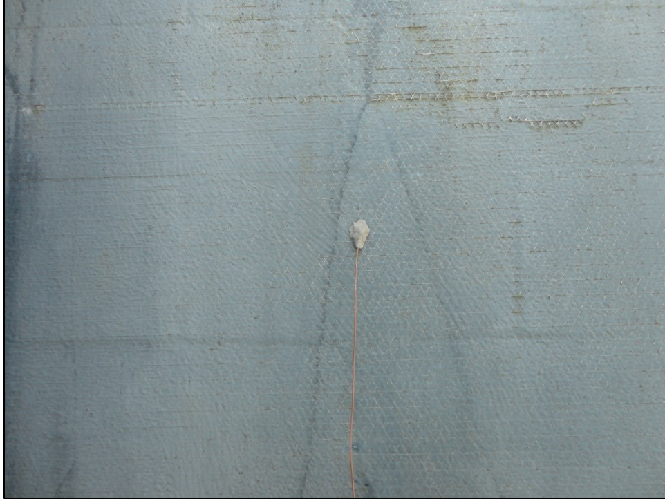
Figure 32: Wall 2 Location 2 Photo (North Side)
