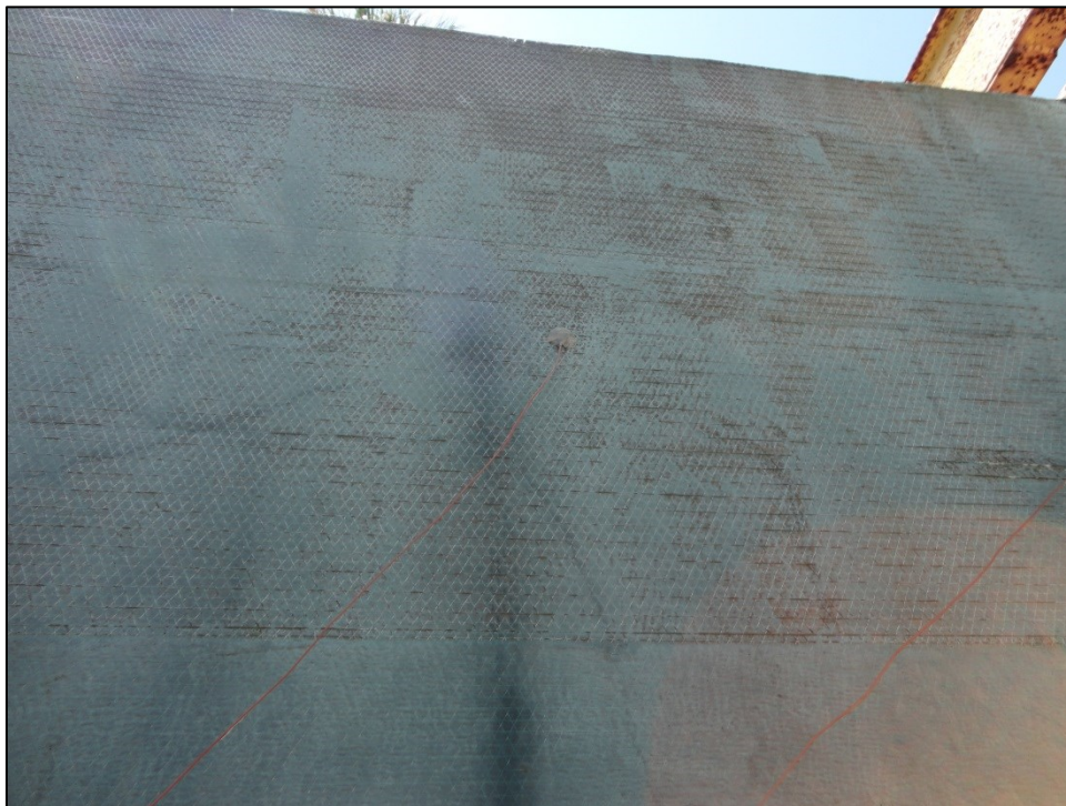
Figure A24: Photo at Location 7 (North Side of Wall 2)
