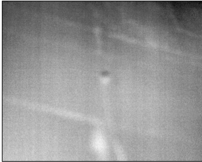
Figure A7: Thermal Image at Location 2 at 10:32 AM (North Side of Wall 2)
