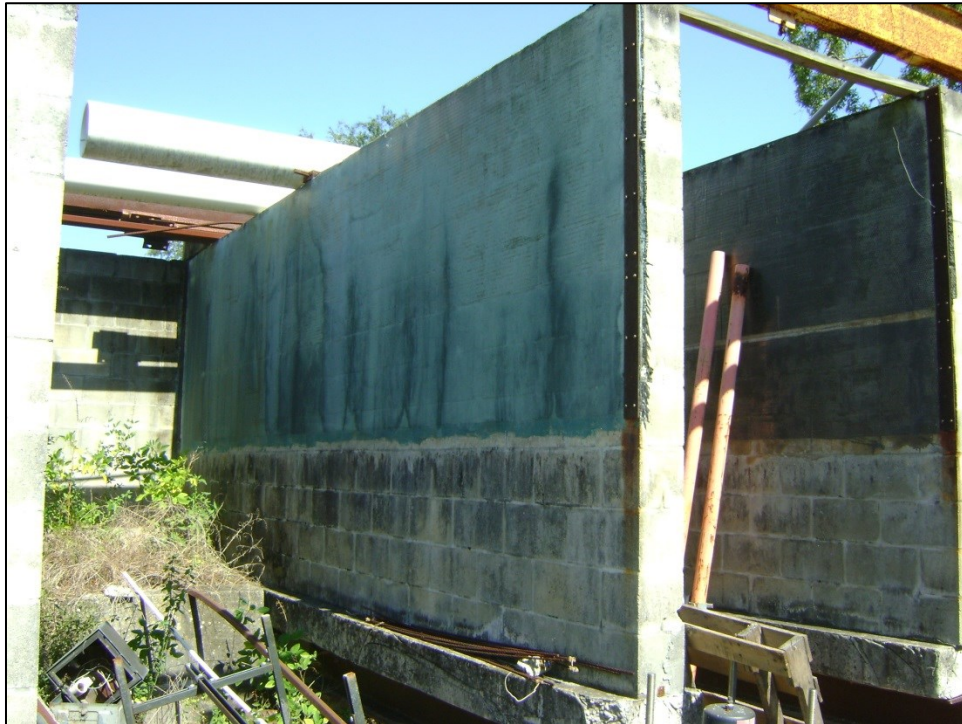
Figure A3: Wall 2
