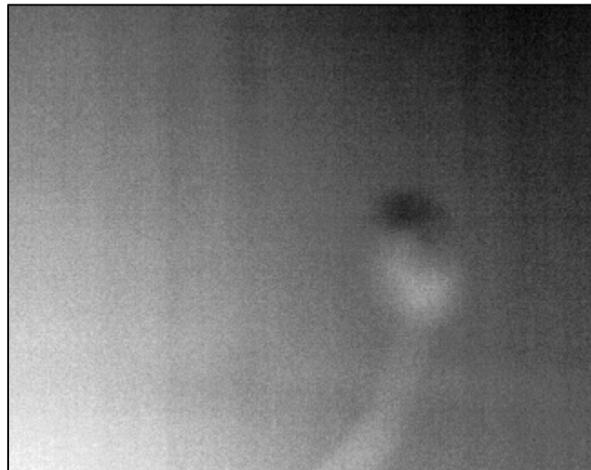
Figure A64: Thermal Image at Location 21 at 1:06 PM (North Side of Wall 2)
