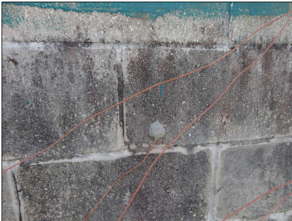
Figure A66: Photo at Location 21 (North Side of Wall 2)
