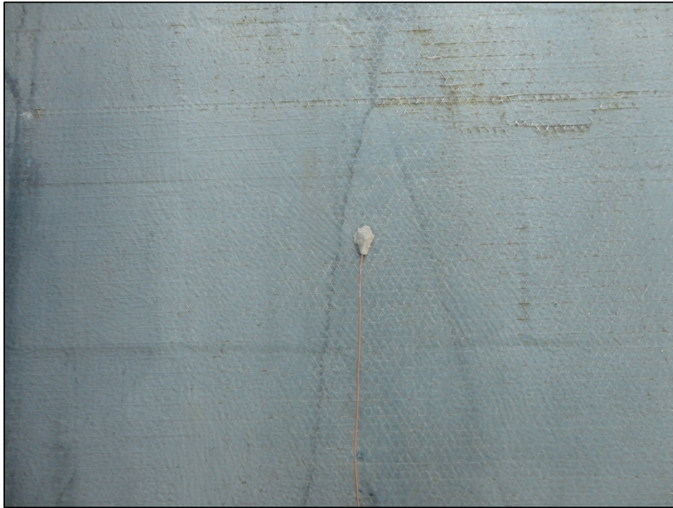
Figure A9: Photo at Location 2 (North Side of Wall 2)
