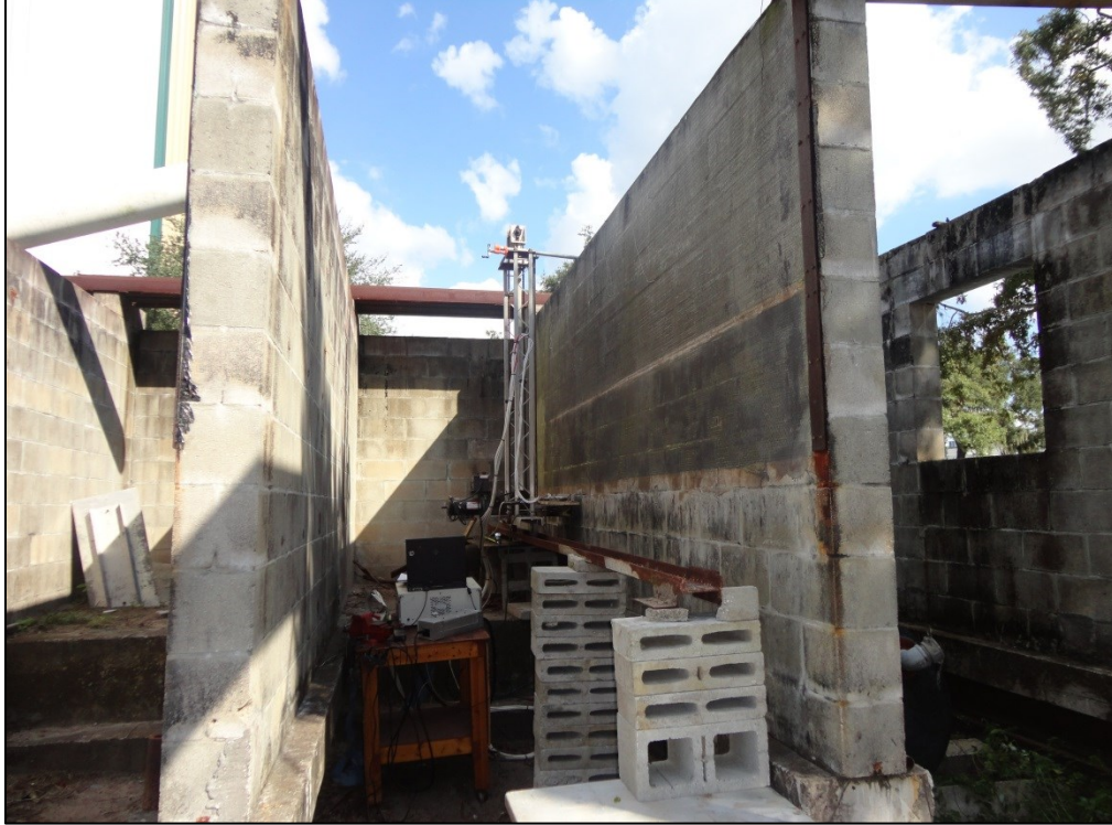
Figure 49: Thermal Scanner Setup on Wall 3
