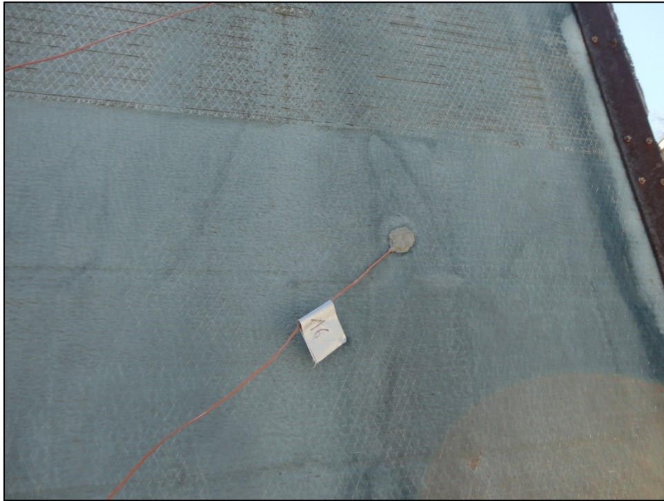
Figure A51: Photo at Location 16 (North Side of Wall 2)
