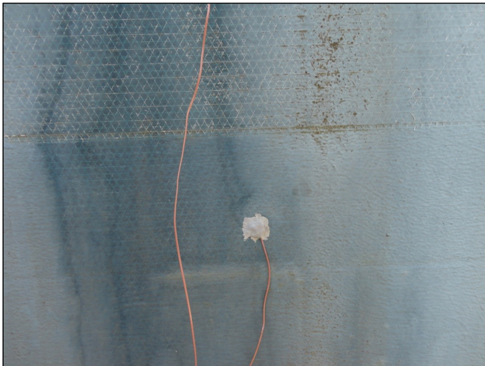
Figure A36: Photo at Location 11 (North Side of Wall 2)
