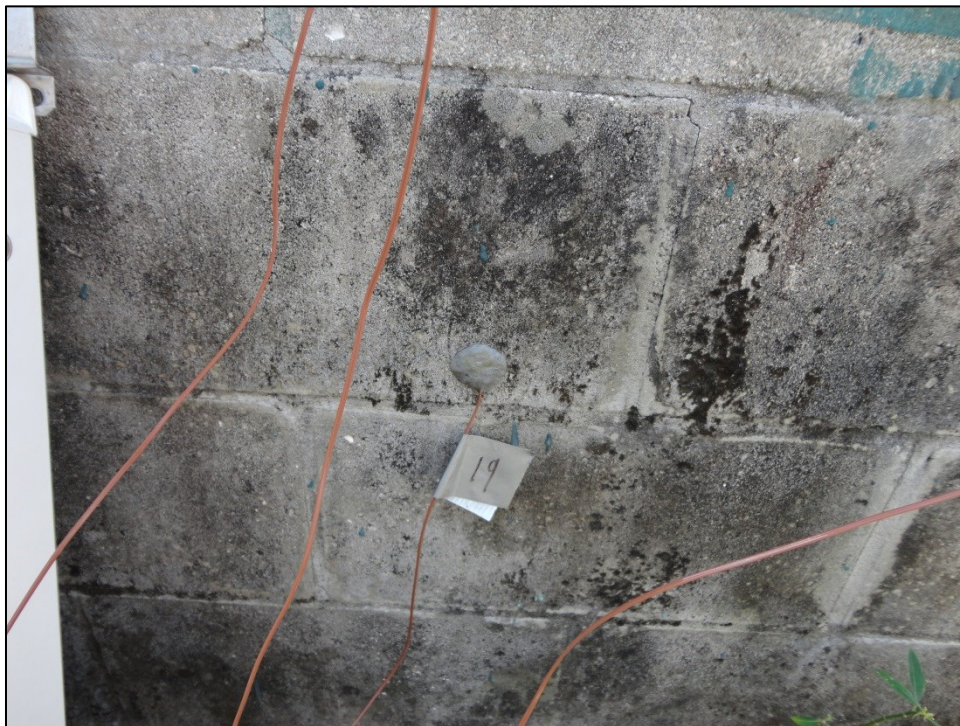
Figure A60: Photo at Location 19 (North Side of Wall 2)
