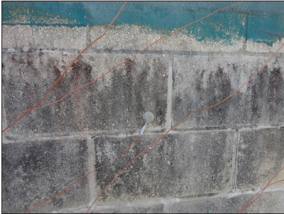
Figure A69: Photo at Location 22 (North Side of Wall 2)
