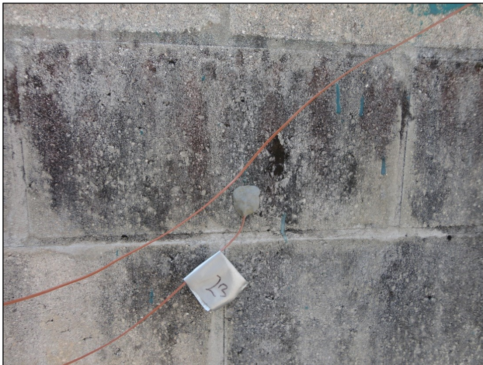
Figure A72: Photo at Location 23 (North Side of Wall 2)
