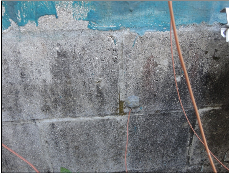
Figure A57: Photo at Location 18 (North Side of Wall 2)
